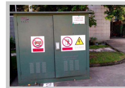
10kV临时一线#2电缆分接箱
